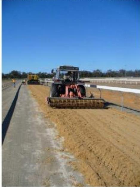
Completing the first lap - the surface is laid on to a conventional road base
