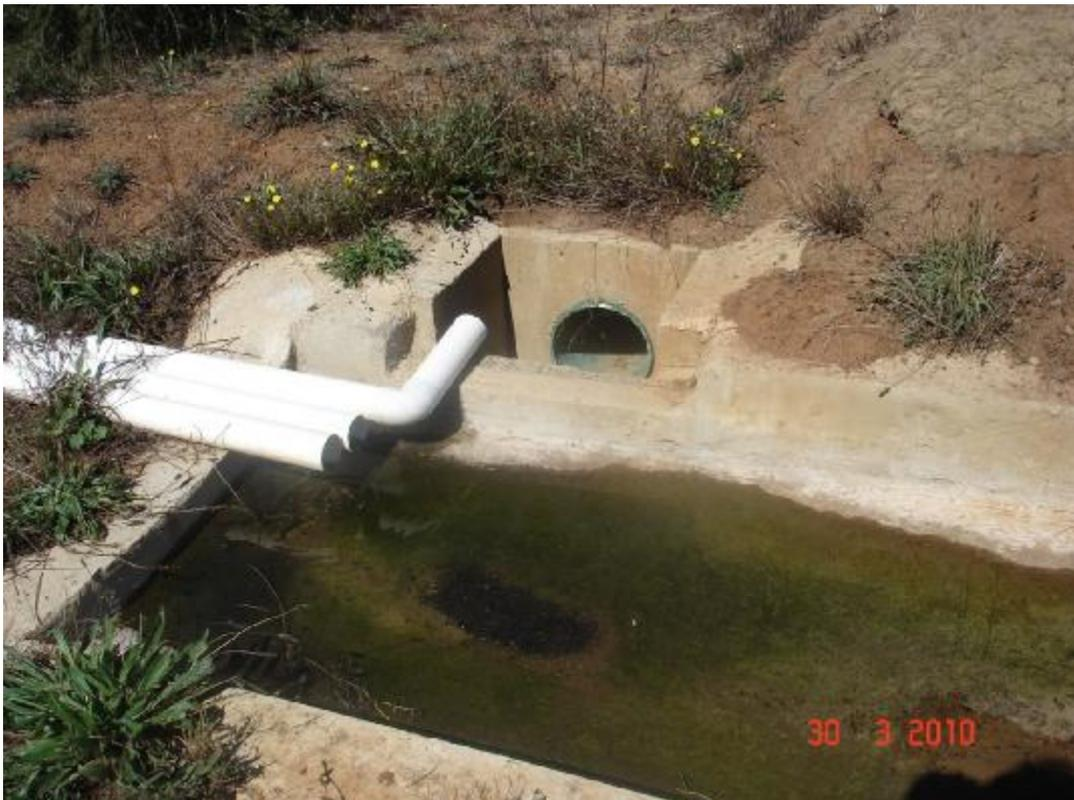
Surge diverter showing spillway which is set at an exact level to prevent stormwater flowing over earth banks downstream.
