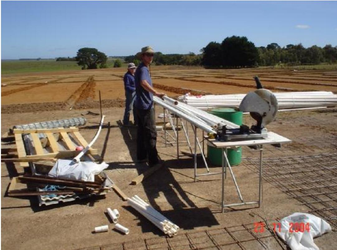
November 2004. Irrigation and drainage/collection networks being fabricated and installed
