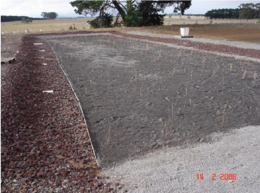
February 2008. *The reed bed has been planted with rhizomes of common reed and inundated to allow the subsurface portions of the plant to develop and produce new emergent shoots.*
