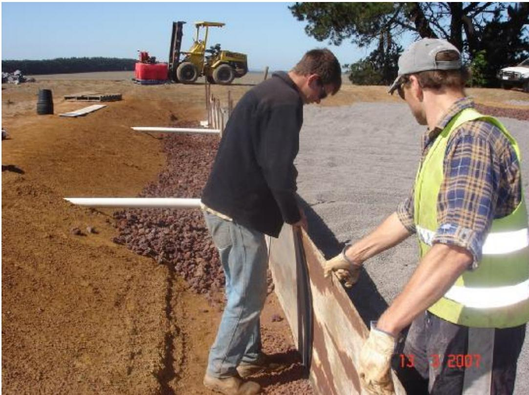
*Installing the inflow manifold to the reed filtration structure*
