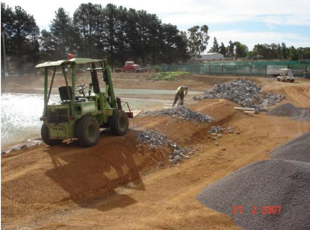
February 2007. Extensive rock walling and beaching in the storage and reed bed areas is being placed to reduce wave action and rain impact erosion to the earth structures.
