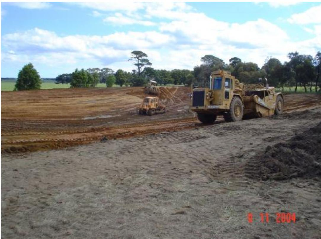
November 2004. Due to site constraints the storages have been constructed to be as deep as possible with the minimum surface area. There was abundant clay on site to line the structure.
