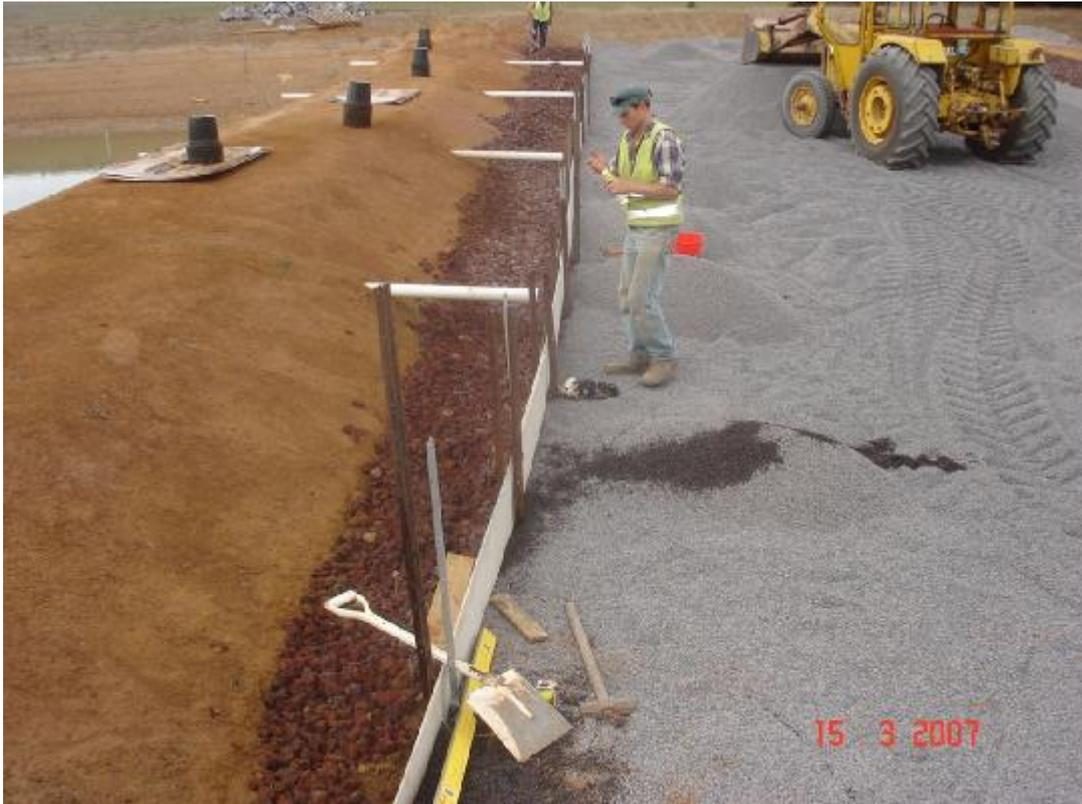
March 2007. *Extensive pipe networks are designed to ensure that the highest level of flow uniformity was achieved through the gravel media.*
