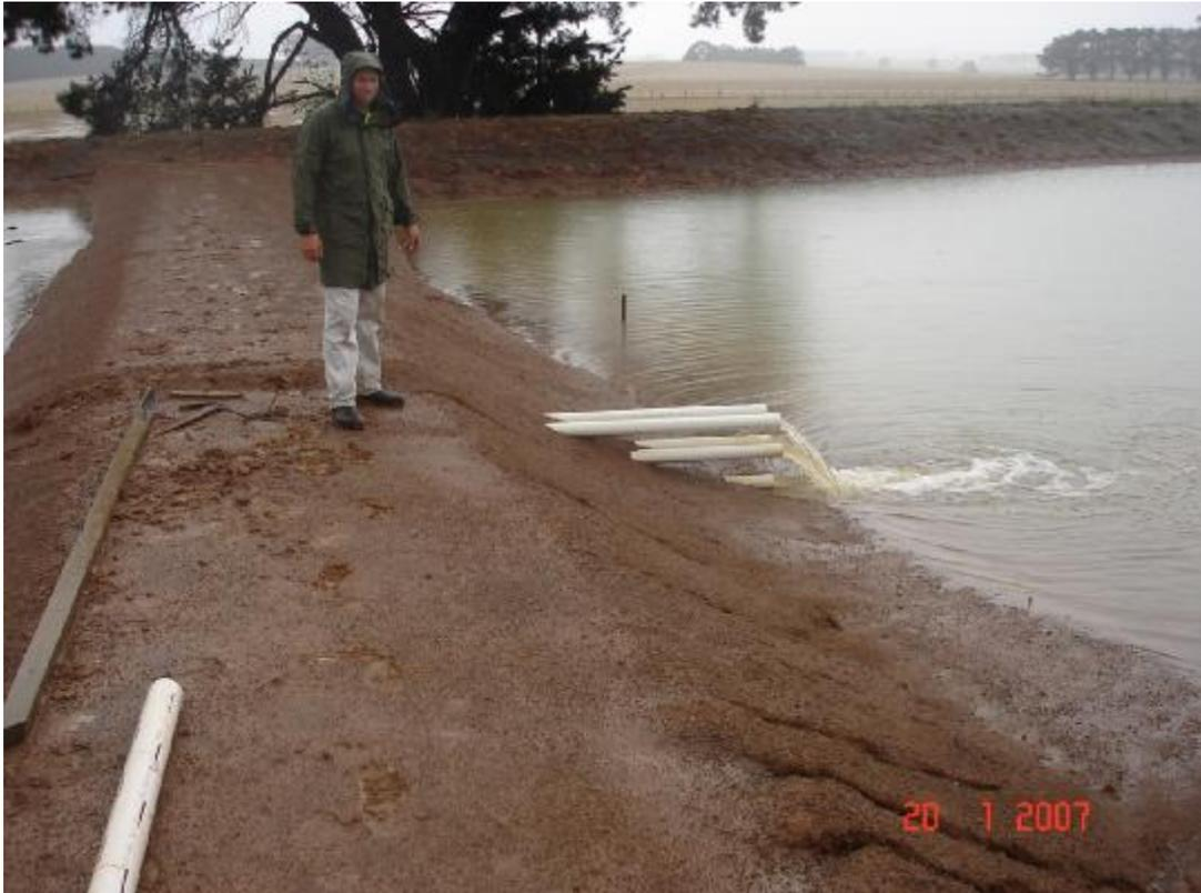
January 2007. A 90 mm in 24 hours rainfall event caused significant damage to the partially completed earth structures
